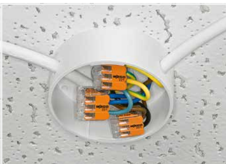
Lighting distribution in ceiling canopy
