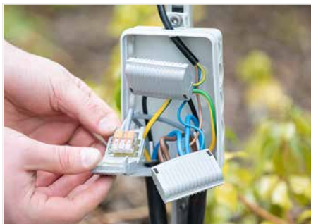
Connecting a bollard light
