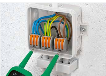
Testing the wired connectors.
