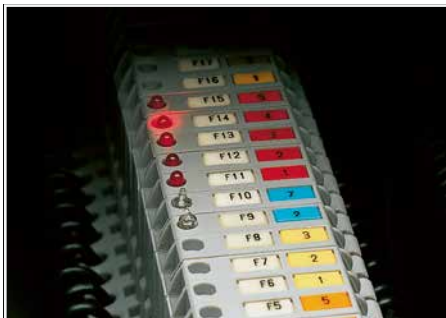
Blown fuse indication by LED or neon lamp
