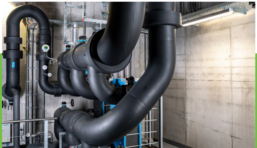
The district heating ducts at the headquarters of IBC Chur
